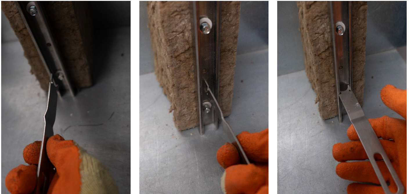
Figure 13 – Installation of wall-ties into retention channel
