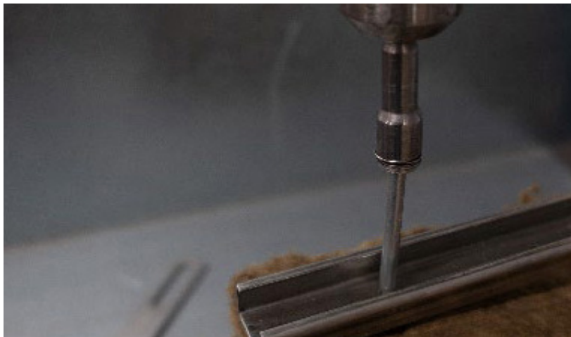
Figure 12 - Installation of fasteners for retention of wall-tie system to concrete or masonry
