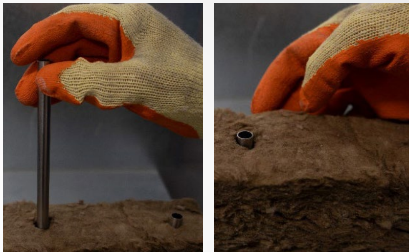
Figure 08 – Installation of anti-compression sleeves
